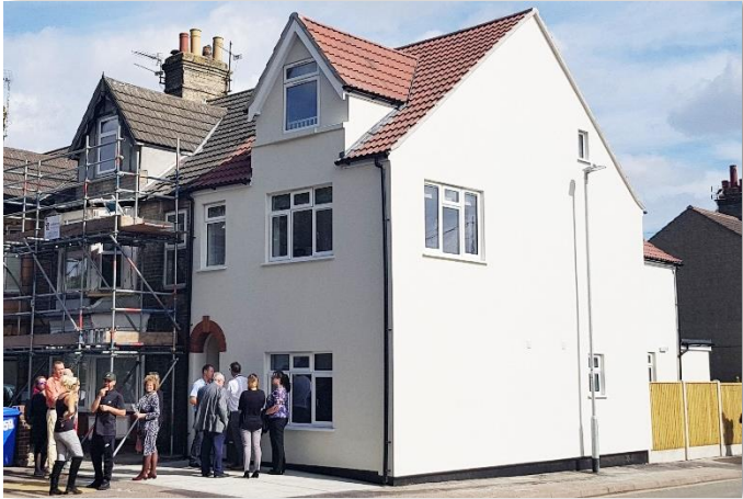
Example of a property in East Suffolk that has been renovated with external insulation applied and rendered. The property was also installed with double glazing to improve energy efficiency and a 6 bike cycle rack to increase the opportunity for sustainable travel.
