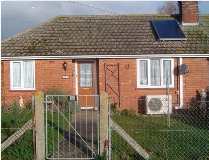
Example of a property in East Suffolk that has installed a solar thermal heating system to reduce the amount energy the property consumes.
