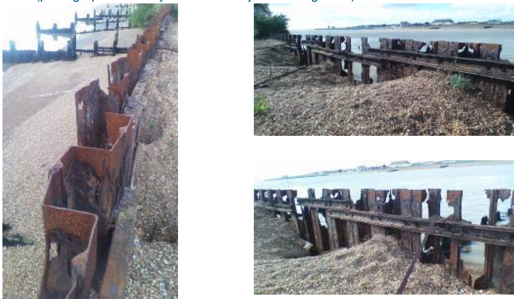
Plate 3.3. Bawdsey Quay Steel Sheet Pile Wall – recent inspection of the central section of wall (October 2016).
